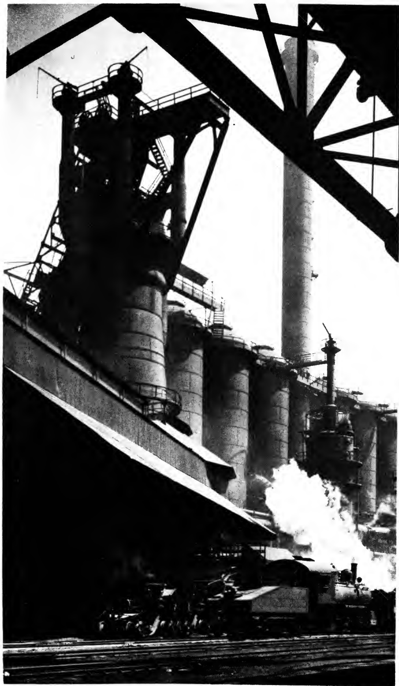
Blast Furnaces, Gary Works
