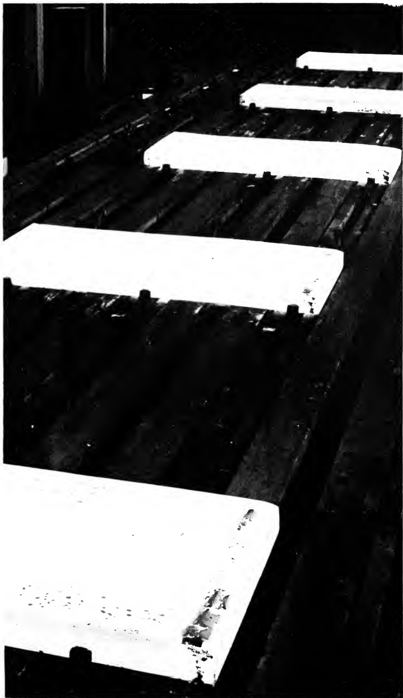
White Hot Slabs Being Conveyed Through the Inland Steel Plant
