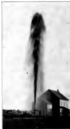
FIG. 1. Town well, Woonsocket, South Dakota; 725 feet deep; yields 1,150 gallons per minute; is throwing a stream 97 feet, under a pressure of 130 pounds per square inch.
