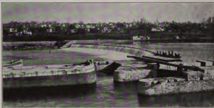
FIG. 7. Canal boats about to enter the locks. A canal very frequently runs alongside a river. Here a dam has been built across the river in order to supply the canal with water.
