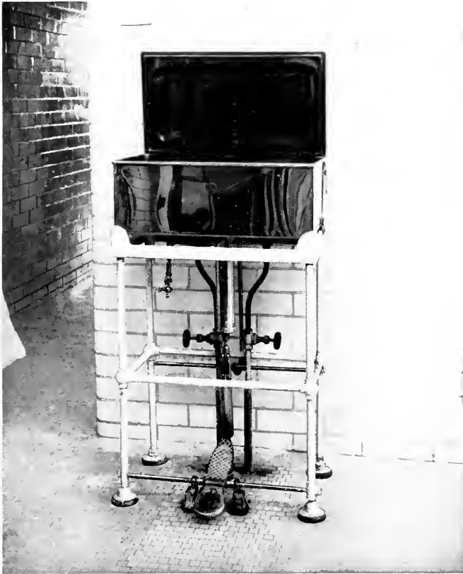
Fig. 1.—Showing instrument sterilizer open. High-pressure steam pipes under the flooring, and entering the sterilizer from below.
