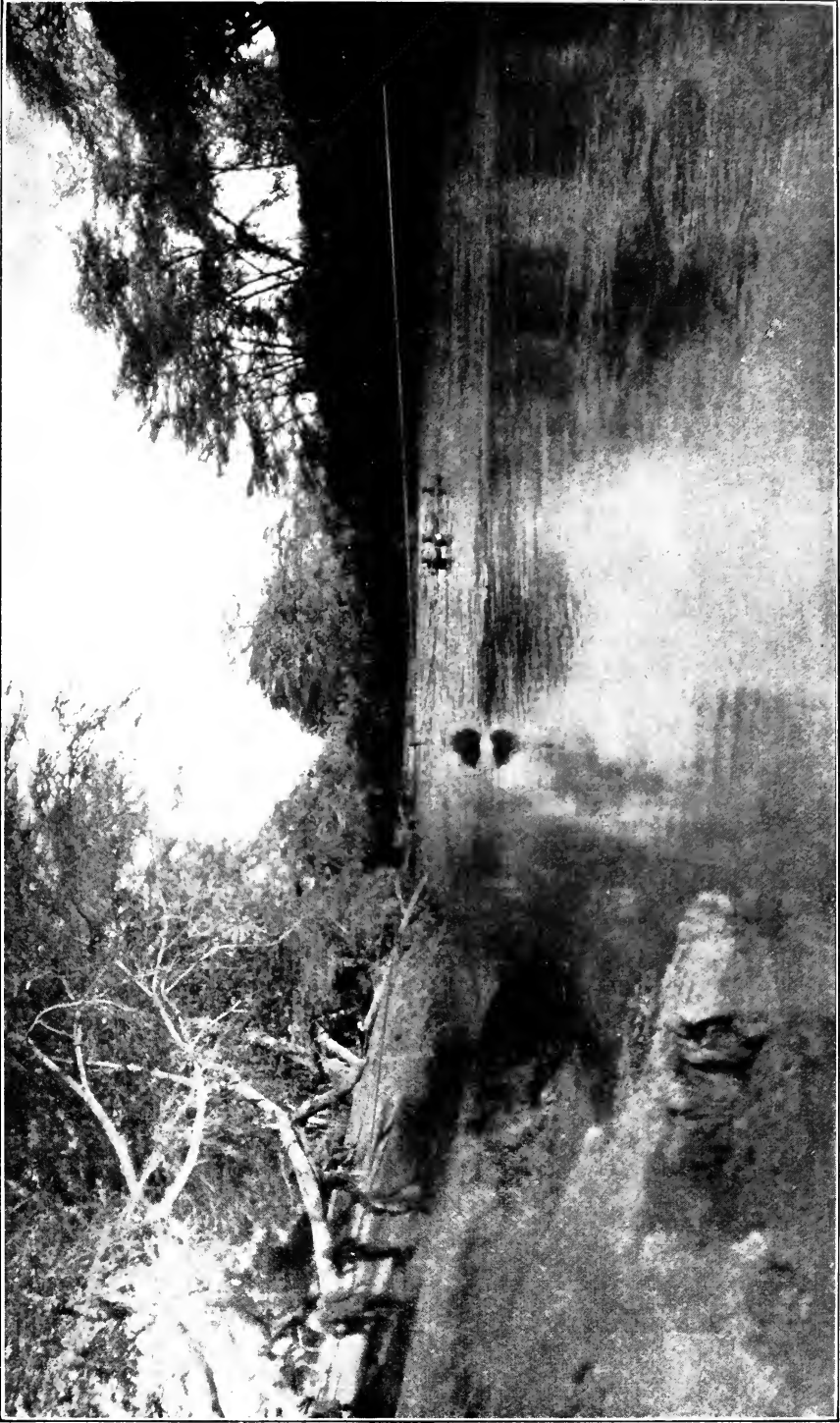
ON THE CABLE WE STRUNG A SNATCH BLOCK AND A LIGHT LINE, AND THUS BY STRINGING LOADS TO THE BLOCK WE PULLED THEM ACROSS
