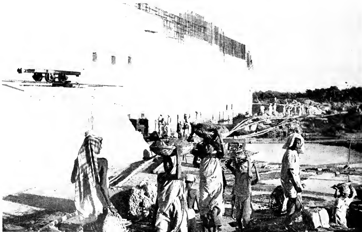
Construction of the Hirakud River dam in India. This multipurpose dam will eventually irrigate almost 2 million acres. The dam is 3 miles wide, with the dykes extending 11 miles. The Indian Government is spending the equivalent of $175 million for this project, and the United States has contributed technical knowledge and earth-moving equipment.
