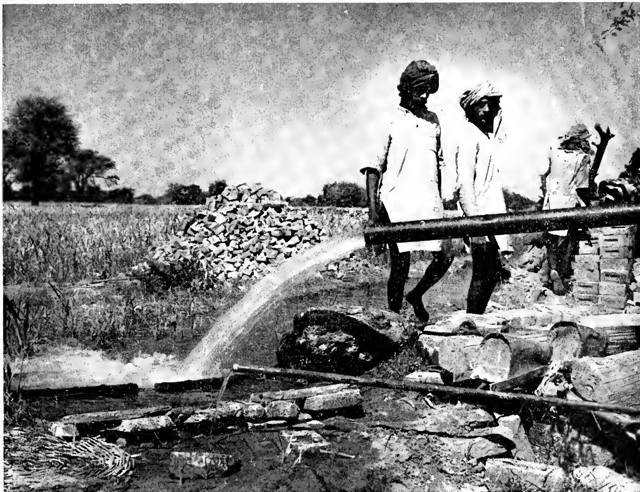
Water for India's campaign to grow more food comes from this new tube well, financed in part by the Indian Government and built with the assistance of American technicians.
