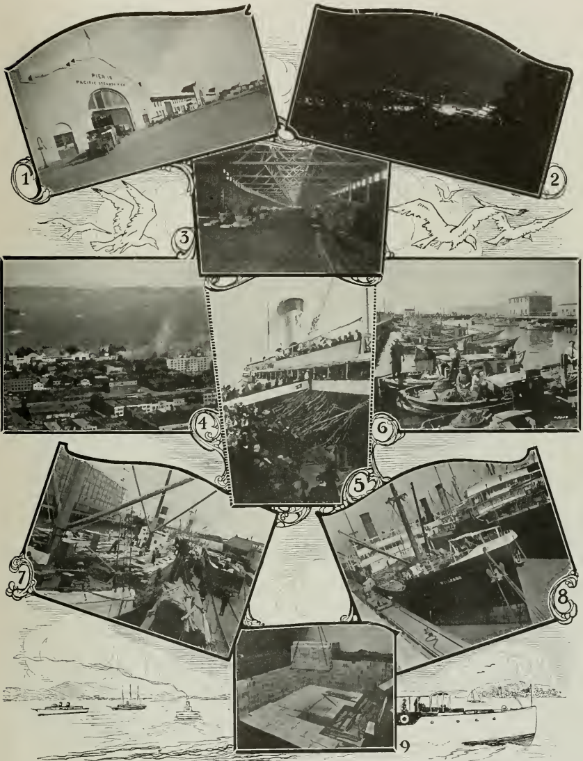
San Francisco's Waterfront is numbered among the world's finest. The accompanying pictures show: No. 1—One of the forty-two modern piers over which pass the great foreign and coastwise trade of the port; No. 2—A night view of the "front"; No. 3—Interior of pier; No. 4—The bay from Telegraph Hill; No. 5—"Sailing Day"; No. 6—Fishermen's Wharf; No. 7—Unloading lumber, China Basin; No. 8—Cargoes for the world; No. 9—A typical cargo of California fruits for Europe.
