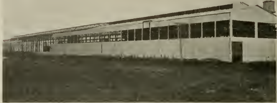
New Addition to the Plant of the Western Pipe and Steel Company, South San Francisco. This building is 1240 feet long.
