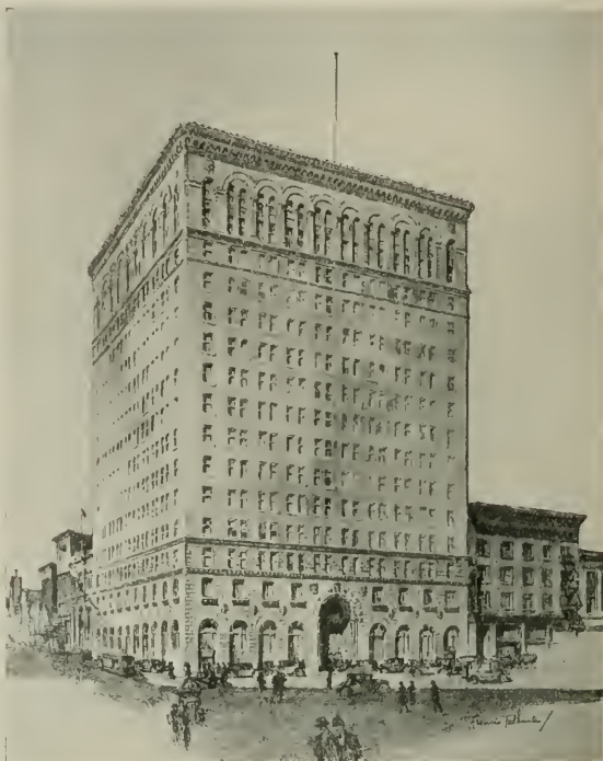
The fifteen-story Financial Center Building now under construction at California and Montgomery Streets
