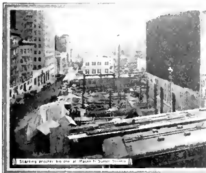
Starting point for one of Market Street buildings
