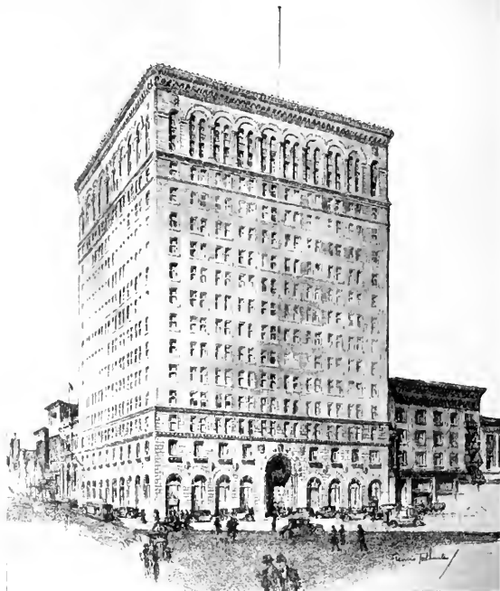
The fifteen-story Financial Center Building now under construction at California and Montgomery Streets.
