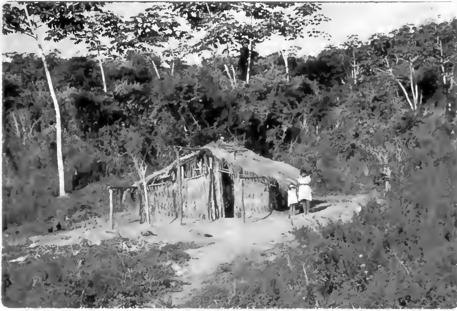
Figure 2.--A "temporary" one year old hut of squatters, Colonia Pindorama, near Penedo, Alagoas, July 14, 1965.
