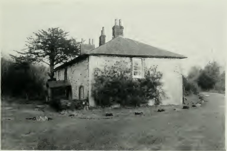
(b) MERSTHAM LIMeworks. LIME COTTAGE FROM WEST.
