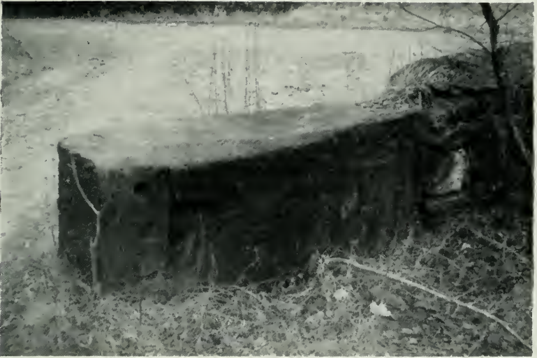
(a) MERSTHAM LIMeworks. BASE OF STEAM ENGINE BUILT INTO WALL NEAR LIME COTTAGE.
