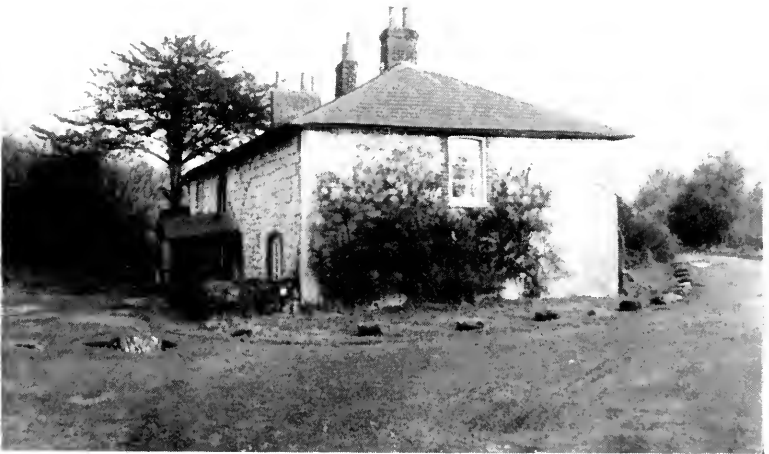
(b) MERSTHAM LIMWORKS. LIME COTTAGE FROM WEST.
