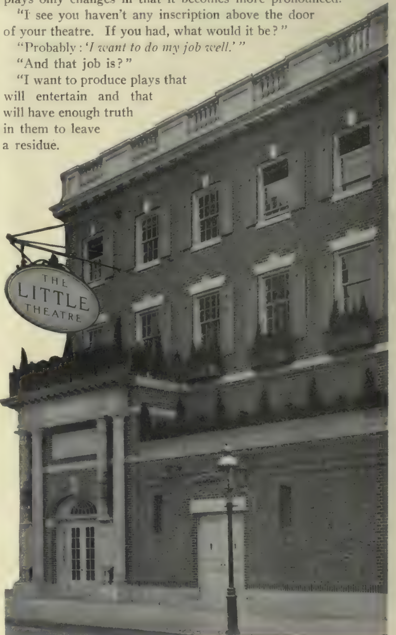
Façade of The Little Theatre, West 44th Street, New York City
